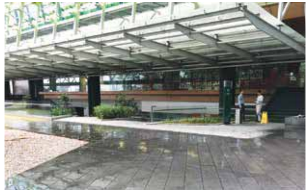
(Image 2: Level 3 Courtyard B)
