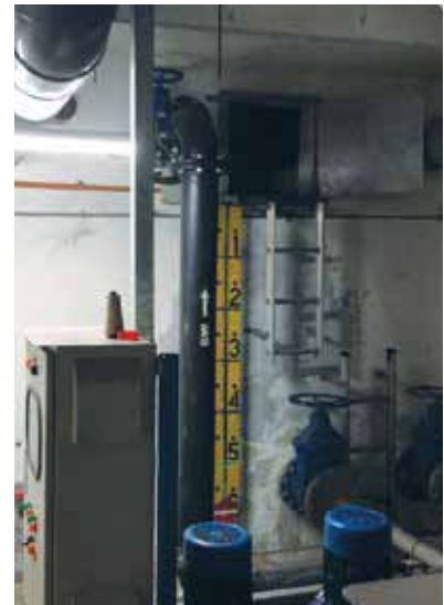
(Image 5: Reinforce Concrete Storage Tank)
