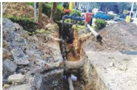
Figure 30: Replacement of underground domestic piping
