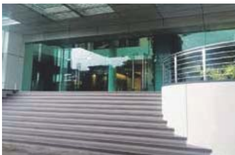
Figure 29: Upgrade staircase with anti-slip tiles
