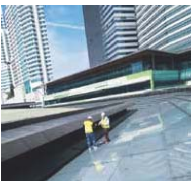
Figure 31: Upgrade of roof rainwater drainage system
