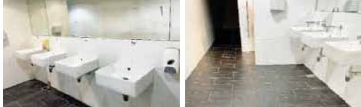
Figure 21-22: Platinum Sentral - toilets before upgrading
