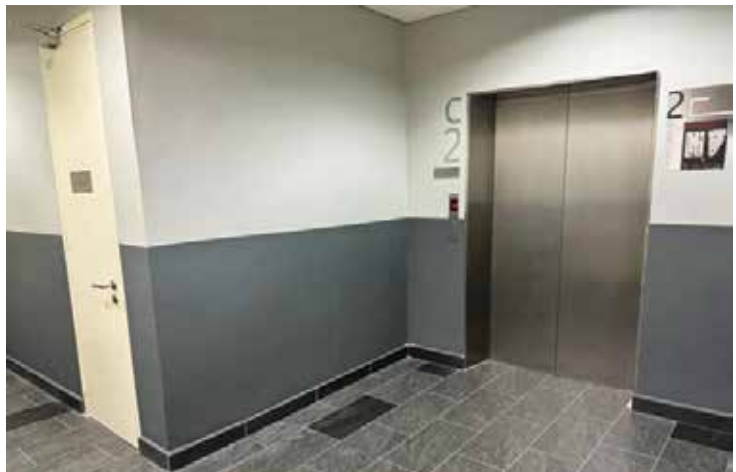
Figure 18: Platinum Sentral - Blocks B & C - after upgrading works
