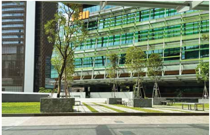
Figure 17: Platinum Sentral - West Courtyard after upgrading works
